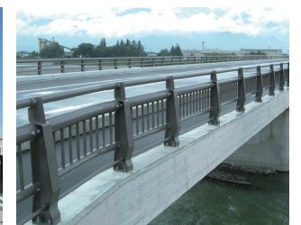
高欄・防護柵 Bridge Railings and Protective Fences
