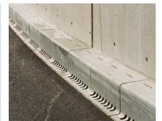
鋼製排水溝 Steel Drain Ditches
